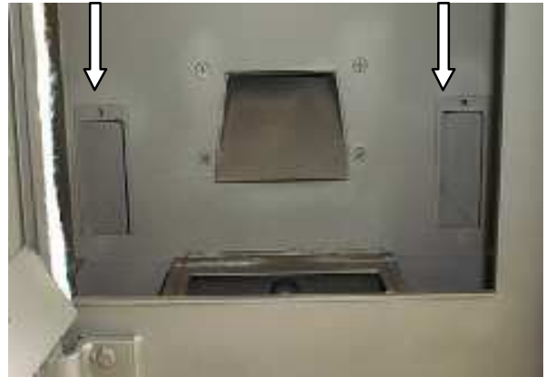
図 19: Lower cleaning aperture, exhaust flues
